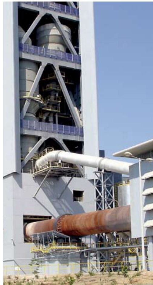
TITAN Cement in Greece is one of the many projects Höganäs Bjuf has supplied with refractory solutions. Photo: FLS Denmark.
